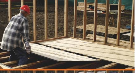
SO WE PUT A NOTCH IN OUR OSB TO DRAIN THE WATER AND CREATED OUR UNIQUE LP TOPNOTCH SUB-FLOORING. IT HELPS PROTECT AGAINST SWELLING AND BUCKLING. AND THAT KEEPS THE PANELS FLAT, THE FLOOR QUIET AND BUILDERS FROM HAVING TO COME BACK FOR REPAIRS. IT'S NOT ROCKET SCIENCE. IT'S JUST SMART.
